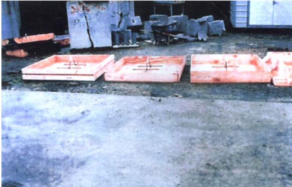
Photo 1. Forms before concrete placement
